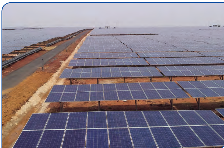
500 MW Solar PV plant of APGENCO in Andhra Pradesh financed by REC.
