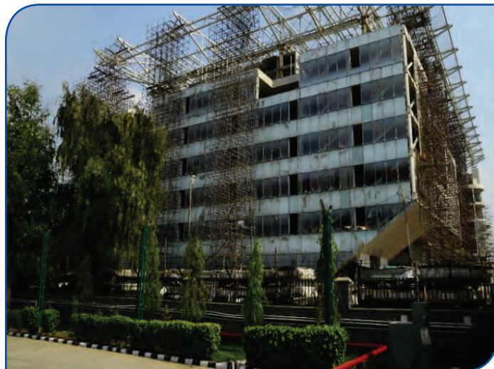
Construction Status of the REC Office at Gurugram
